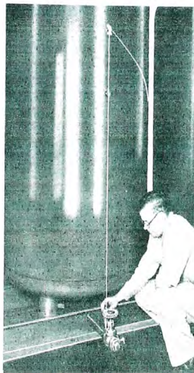
Fig. 3 Plumbing of Breaker
