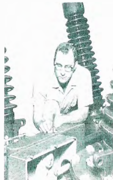
Fig. 13 Method of Measuring Lift Rod Clearance
