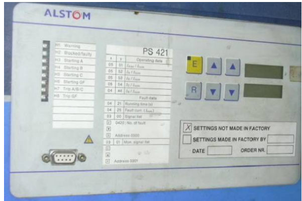
RELE PS421 (Alstom) Autónomo
