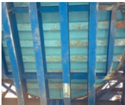
Semi-Supported Tank Bottom on End-User Supplied Supports
