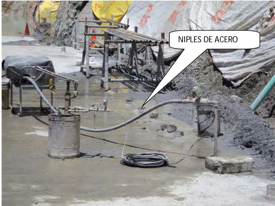
Fig. 2-29:Niples instalados
