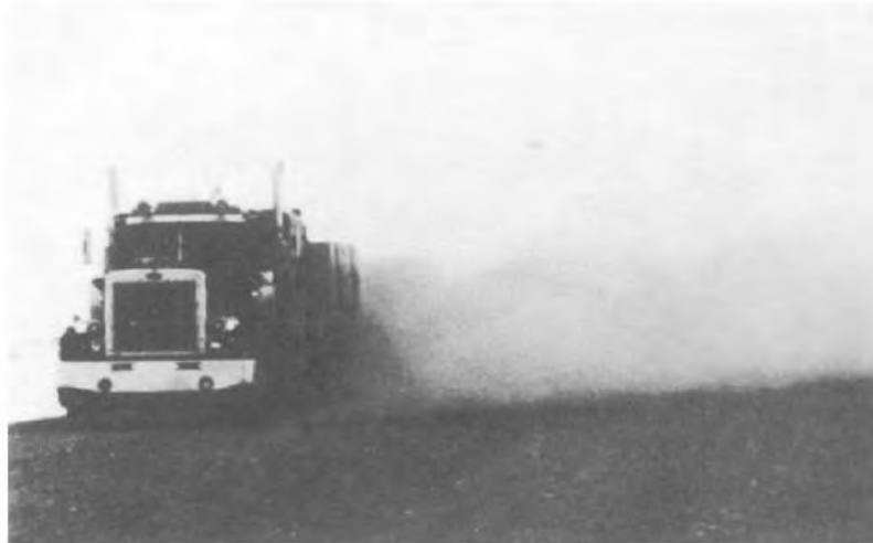
Figure B-8. High severity example of dust.
