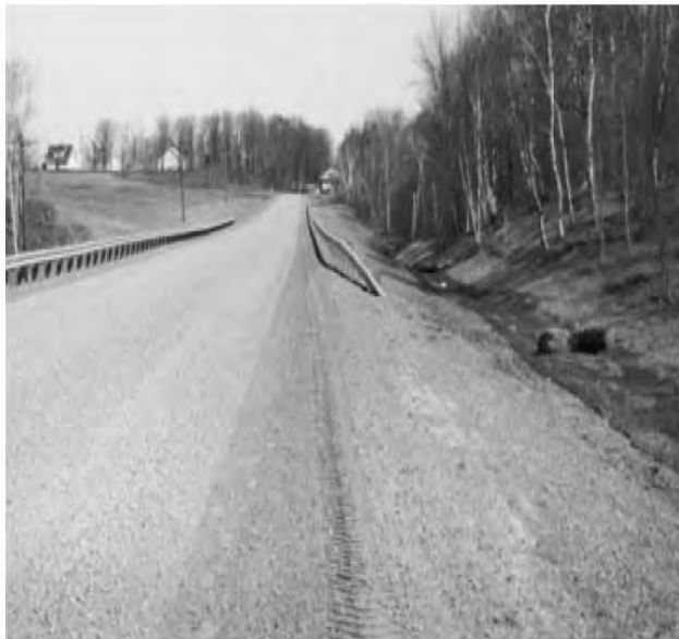
Partial drainage. Ditch and new culvert being added on left. Little or no drainage on right.
