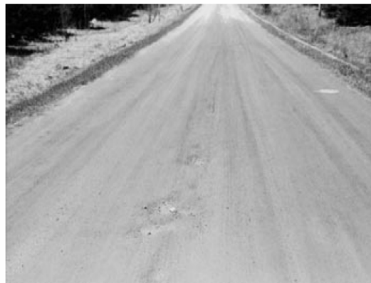
◀ Small, isolated potholes. Routine regrading should eliminate them. ▶ Series of moderate potholes require scarification and regrading.
