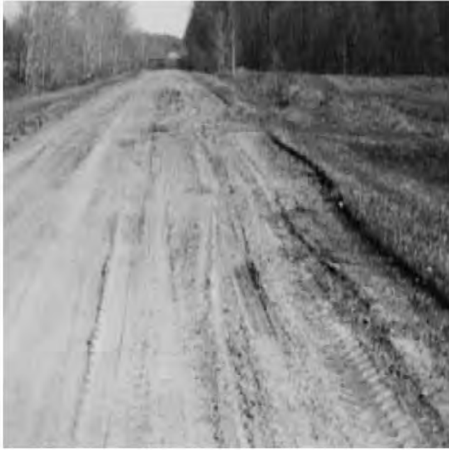
▲ Poorly graded crown traps water causing it to run down center of road.
