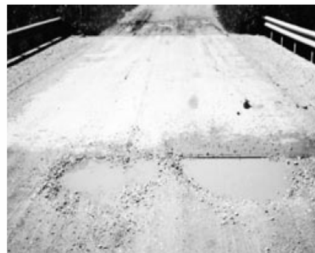
◀ Small, isolated potholes. Routine regrading should eliminate them. ▶ Series of moderate potholes require scarification and regrading.
