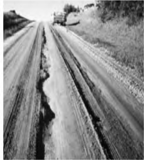
▲ Poorly graded crown traps water causing it to run down center of road.
