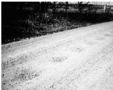
▶ Potholes at bridge may require scarification and hand patching. Gravel and debris should be cleaned off bridge deck.
