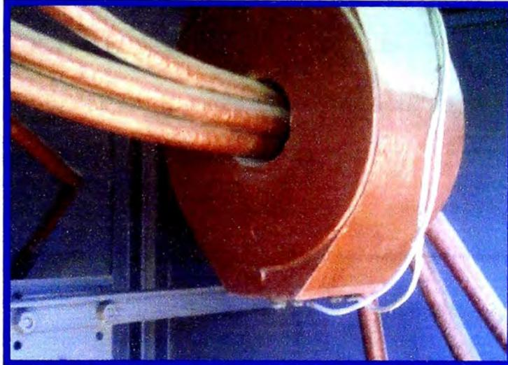
**Fig. 15 Transformador Toroidal**
