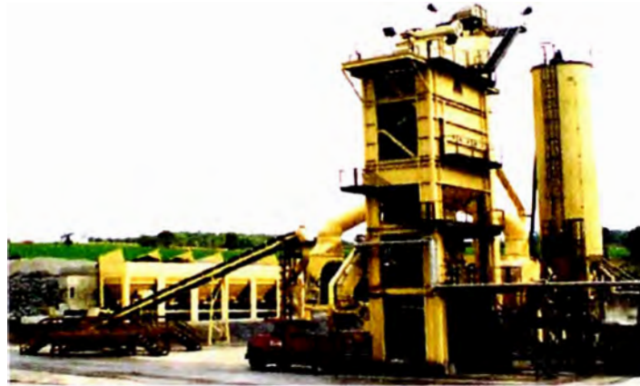
Foto 1.97 Batch plant ASTEC
