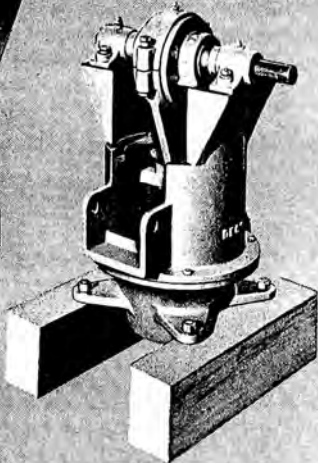
3" DENVER LOW HEAD DIAPHRAGM PUMP
