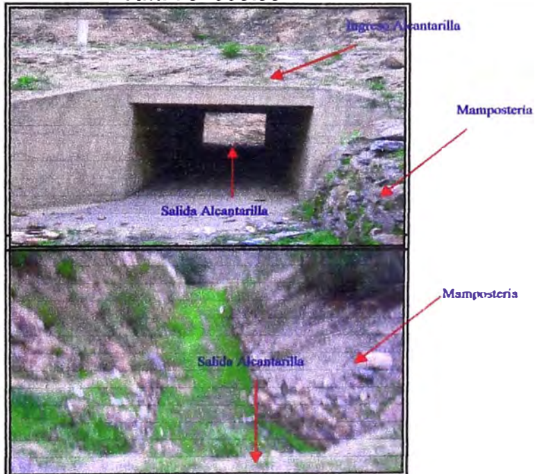
Alcantarilla N° 09 Km. 70+660.00
