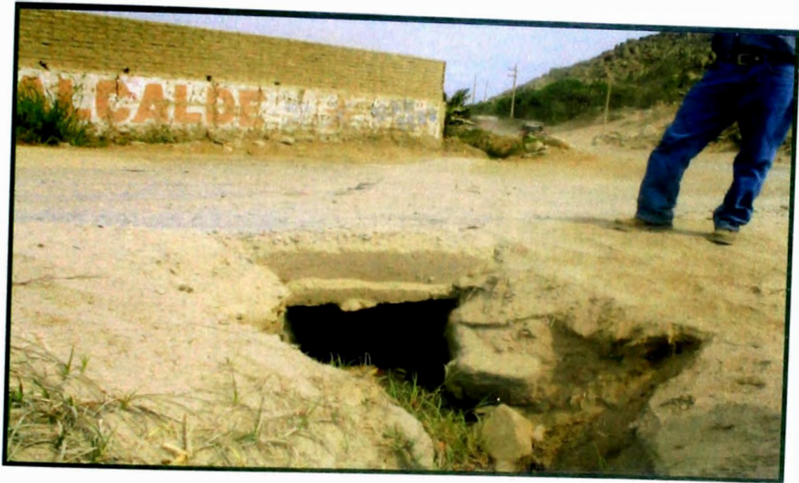
ALCANTARILLA: KM. 10+760 (TRAMO – I)
