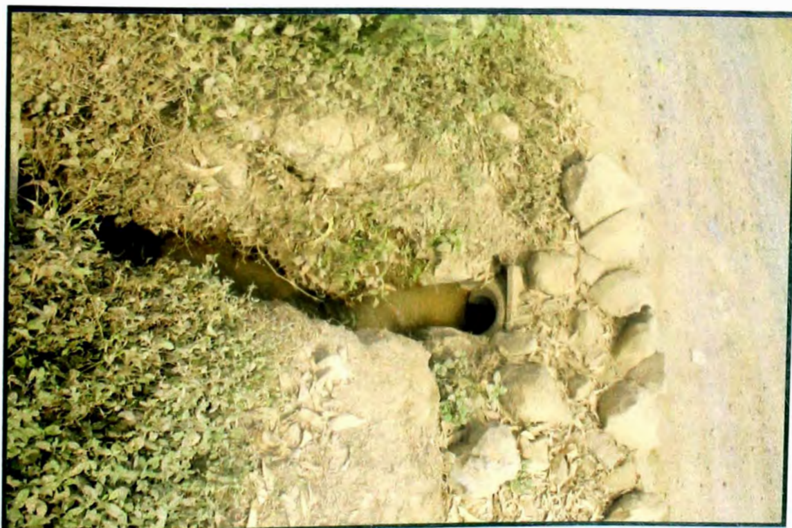
ALCANTARILLA: Km. 10+103.40 (TRAMO – I)
