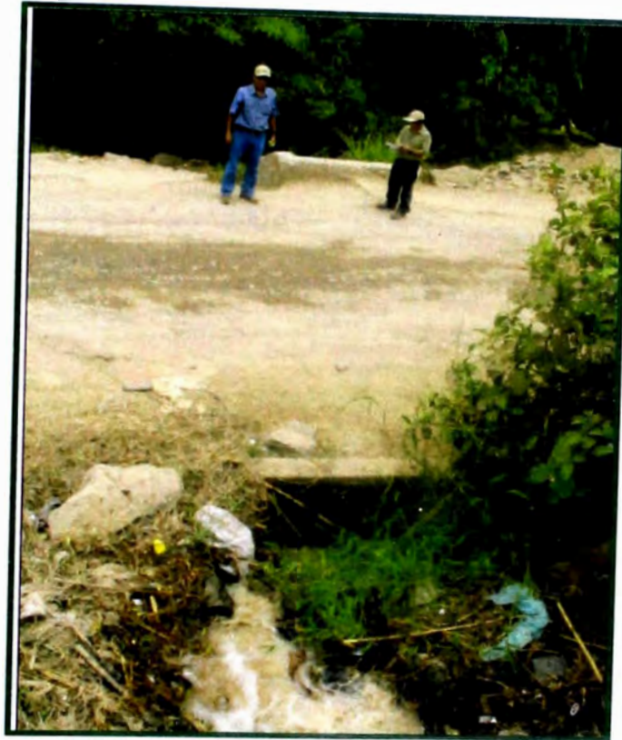
ALCANTARILLA: KM. 9+344.10 (TRAMO - I)
