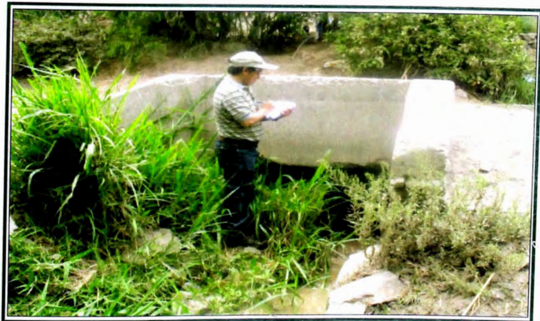
ALCANTARILLA: KM. 0+370.25 (TRAMO - II)
