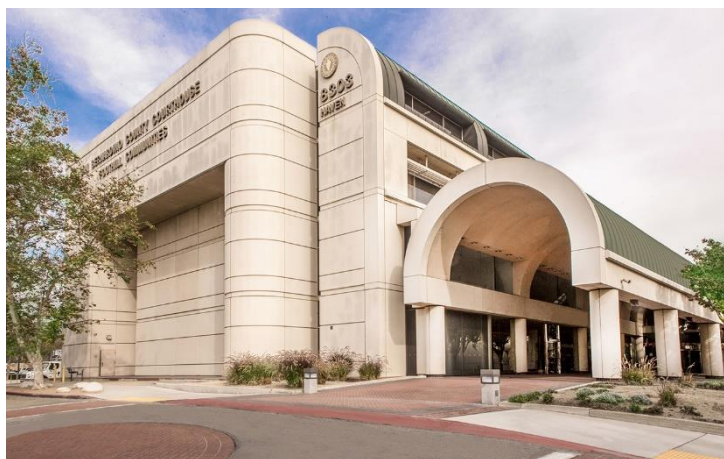
Figura N° 1.5 Foothill Communities Law and Justice Center, EE.UU. (Fuente: http://angelescontractor.com )
