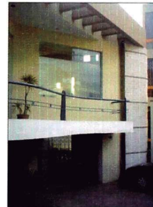
VISTA BALCON EXTERIOR
