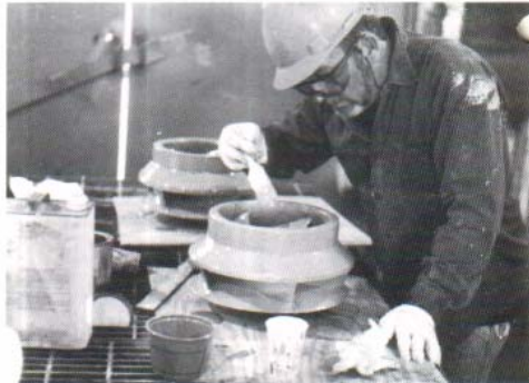
3. Applying Belzona® Superglide.
