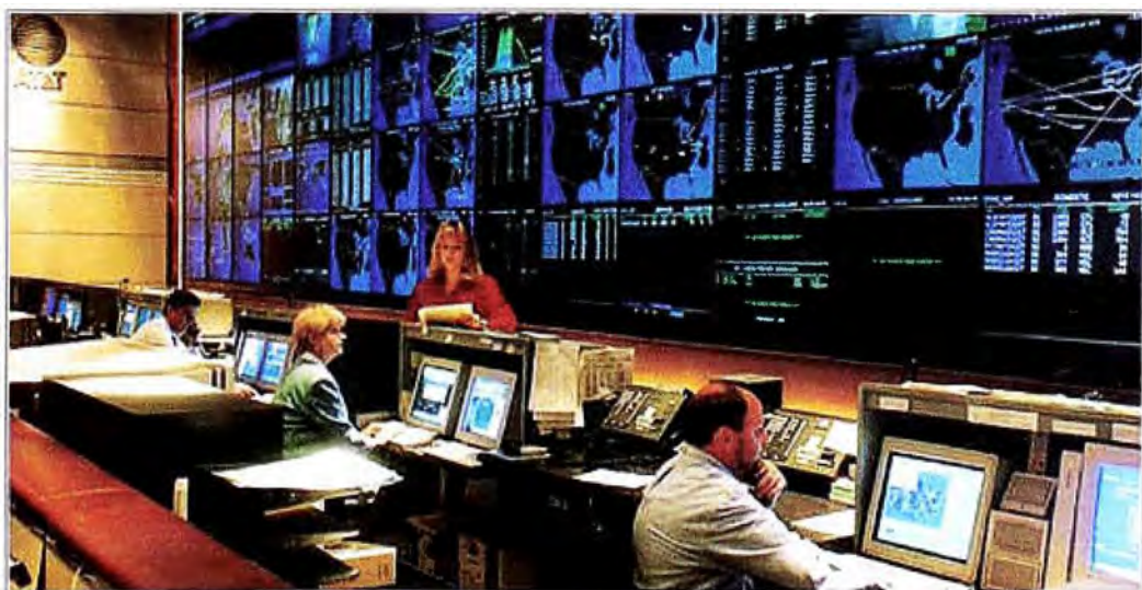
Figura 3.33. NOC Network Operation Center
