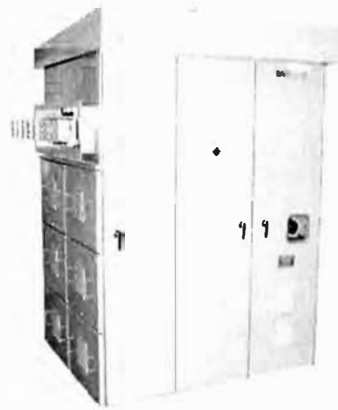
Fig. 5—External View of 6,000-kW Eco-rectifier. An external view of the eco-rectifier that dispenses with materials which cause global warming is shown.
